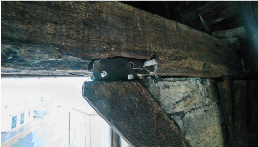
Damaged oak beam visible in 'FPT virtual tour' - Source: Friends of York Walls
