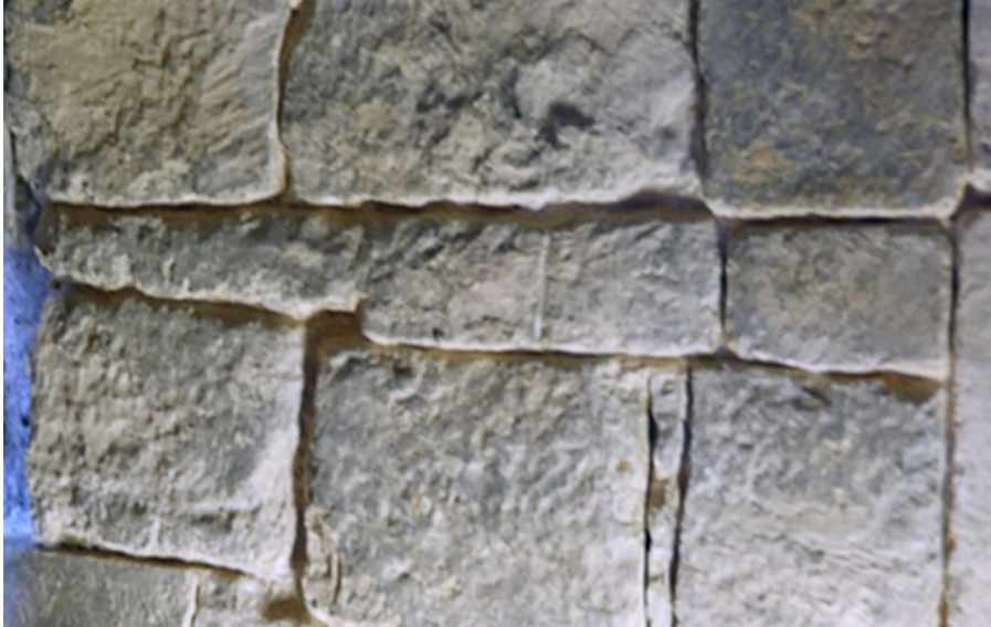
During trial: cement mortar chipped out – Photo: Baz Jones
