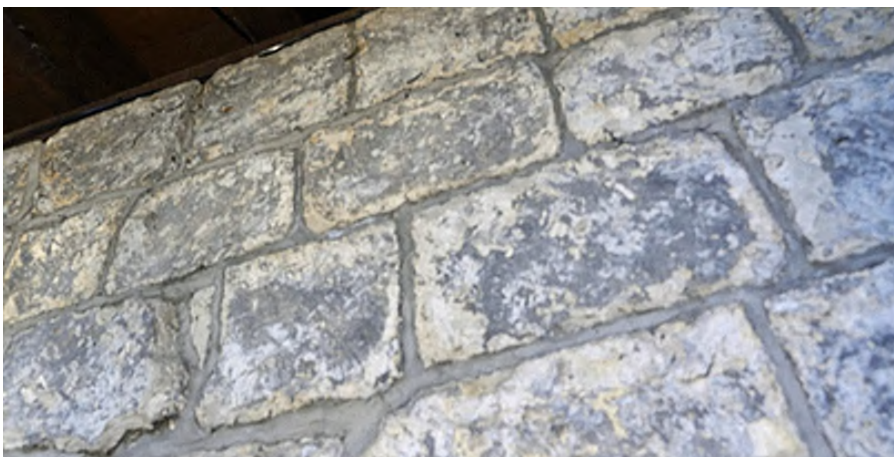
Before trial: showing cement mortar – Photo: Baz Jones
