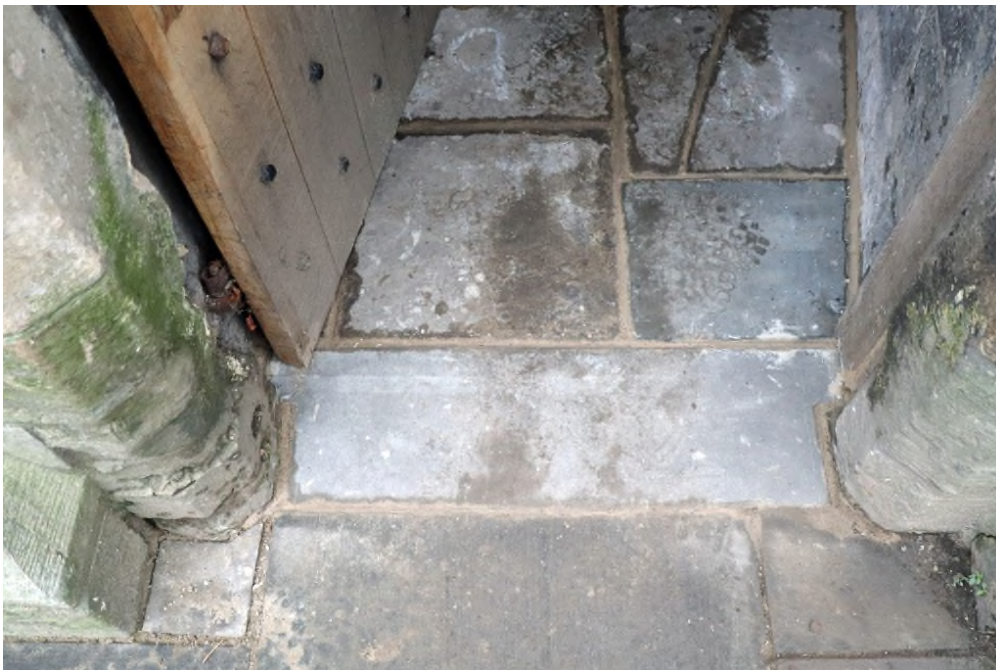
The re-laid Door Sill - Photo: Alan Fleming
