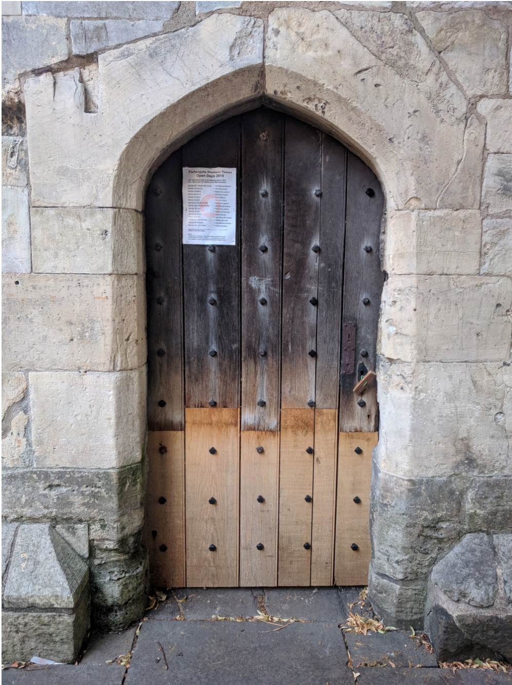
The New Door - Complete with Studs - Photo: Sam McDermott
