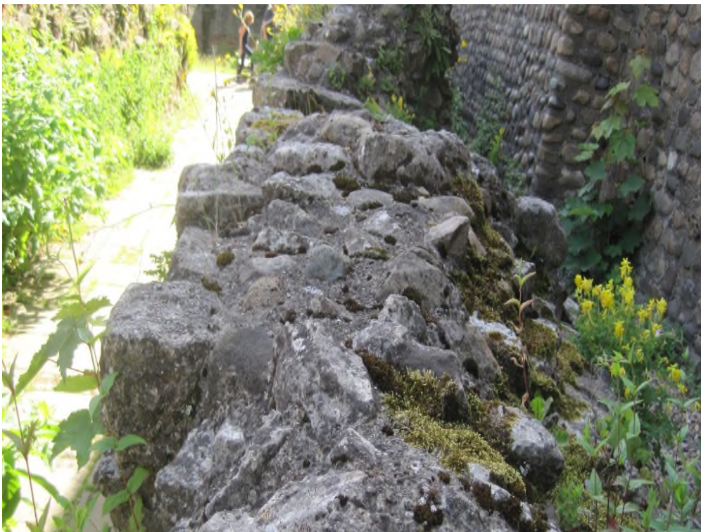
Hard Topping. - Photo: Simon Mattam
