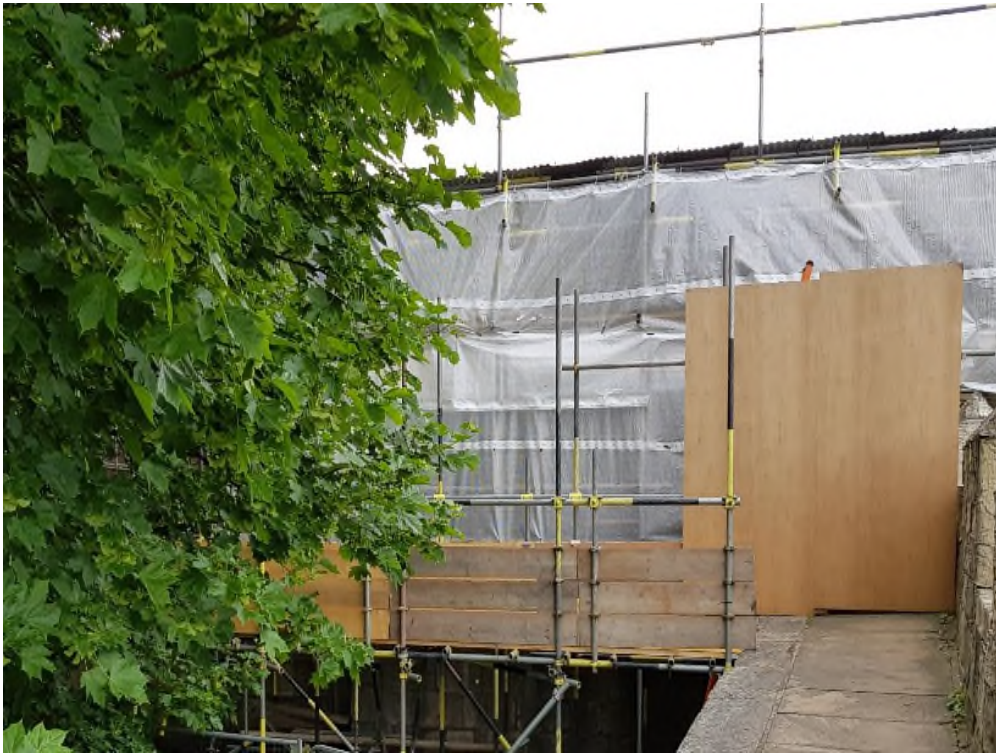
Tower 39 Repair Board - Photo: Richard Hanage
