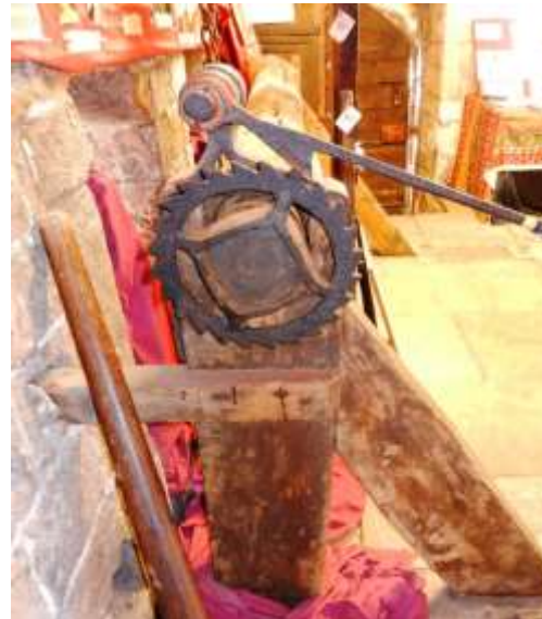
Portcullis lifting winch in Monk Bar
