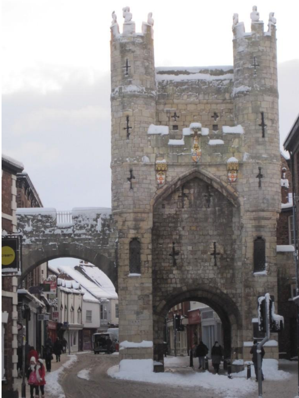
Front of Monk Bar: signs of serious –and less serious– defence. (SM)
